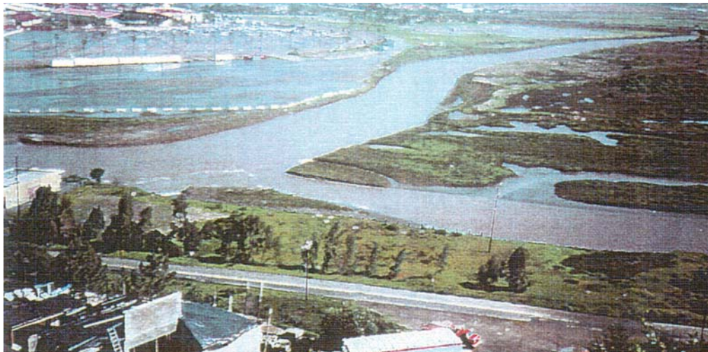
Figure 16. Flooding in the South Lot (photograph by Alice Goodkind). (1995)
