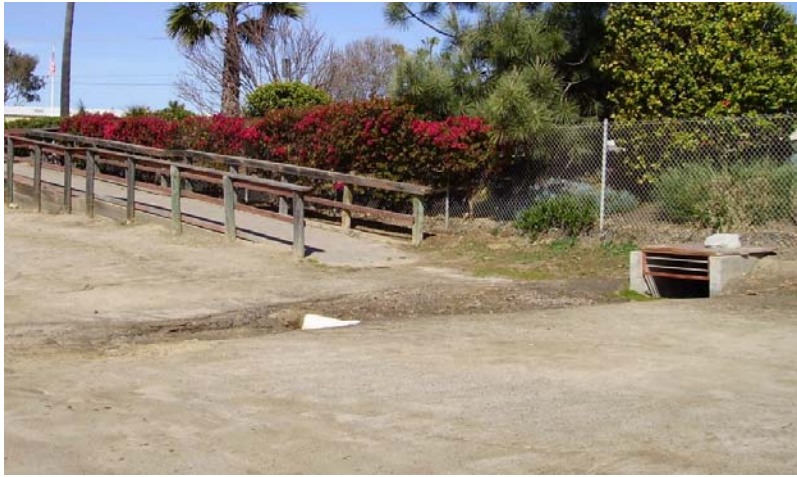
Figure 9. What is the source of the water in the wetlands? Water comes from many sources. The obvious natural sources are a combination of rain and tidal influx. This photograph shows influx of water into the South Lot from the asphalt lot west of Jimmy Durante Blvd.
