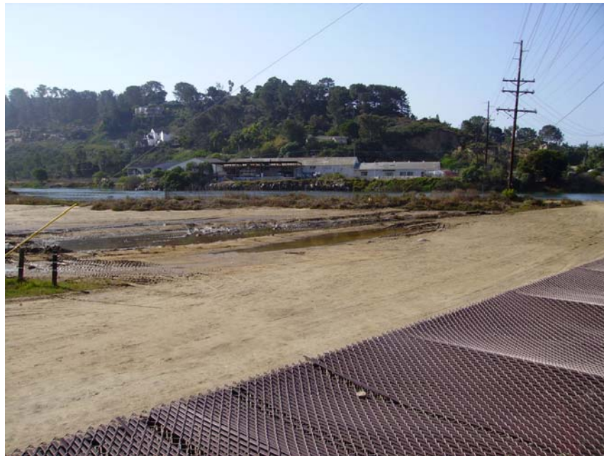
Figure 6. Up-stream from the gate (see Figure 3), a basin had developed around the drainage ditch. As the water flows out, it carries away sediments and enlarges the basin over time. Evaporation leaves white salt deposits. (September 12, 2005)
