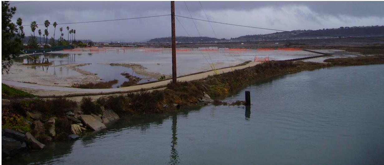
Figure 8. This view, taken from the Jimmy Durante Bridge, shows the respective locations of the two discharge points, the culvert, west of the telephone pole (see Figure 4), and the breach on the right (see Figure 6). (February 19, 2007)
