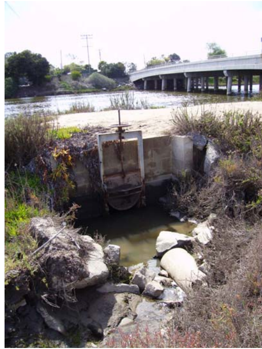
Figure 5. Where does the water in the South Lot go? Some of the water evaporates, some of it percolates in place, and some flows into the San Dieguito River. Water is discharged into the San Dieguito River at the Southwest end of the South Lot through a culvert installed by Fairgrounds personnel. A manual valve gate controls flow. (Left) Gate closed. (Right) Gate open.
