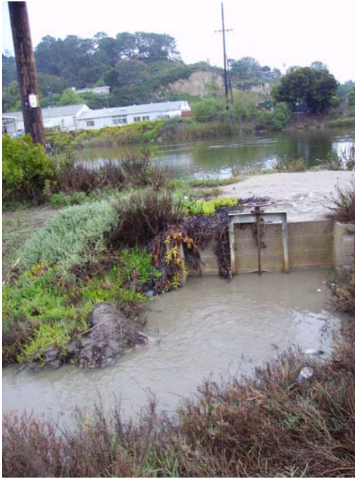
Figure 5. Where does the water in the South Lot go? Some of the water evaporates, some of it percolates in place, and some flows into the San Dieguito River. Water is discharged into the San Dieguito River at the Southwest end of the South Lot through a culvert installed by Fairgrounds personnel. A manual valve gate controls flow. (Left) Gate closed. (Right) Gate open.
