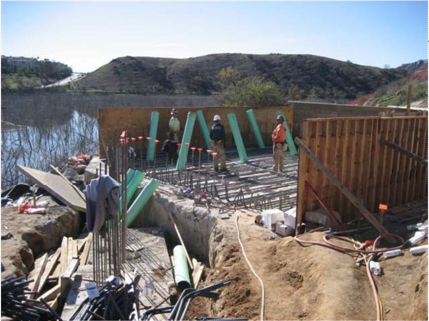
NORTH ABUTMENT CONSTRUCTION
