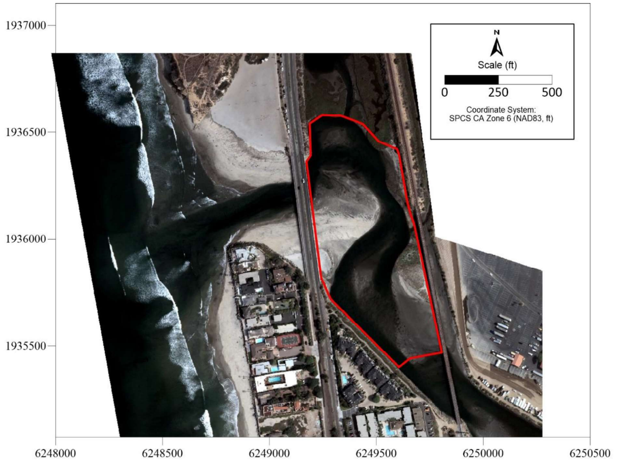
Figure 4. San Dieguito Lagoon Inlet. Red polygon shows area of sand accumulation between Highway 101 and the Railroad Bridge used for calculation of sand volume.
